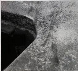
Here's a close up of the corner of the grille opening (left front side). You can see a small spot of significant blast damage at left front grill opening. Typically, this damage only occurs in tight quarters (although I've had a complete panel destroyed during the soda blast process, and it was due to operator incompetence—Ed).
